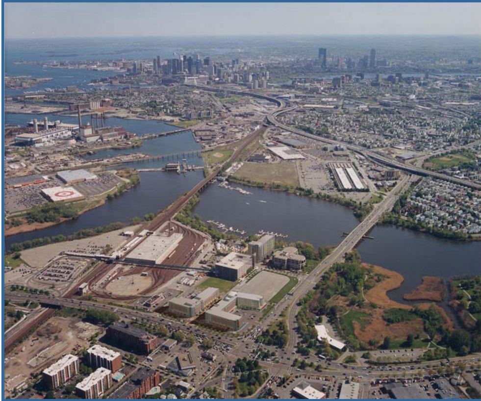
Site for Station Landing by Orange Line on Mystic River National Development
