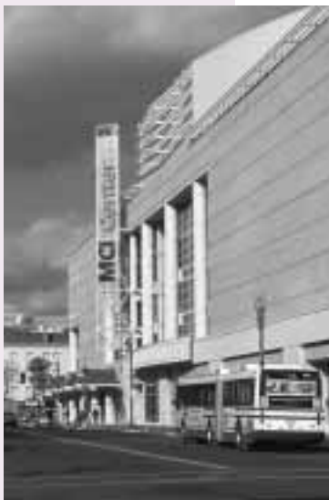
The MCI Center started a development boom in its downtown Washington, D.C., neighborhood.
